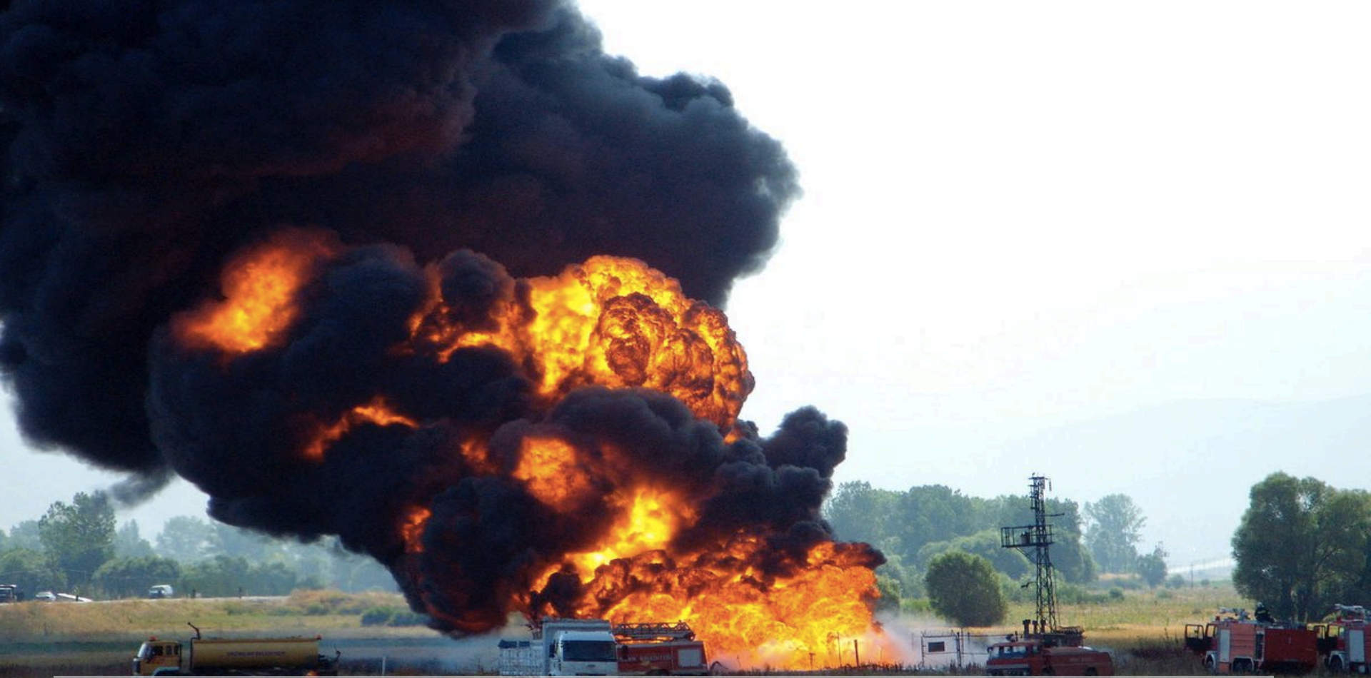
BTC Oil Pipeline
